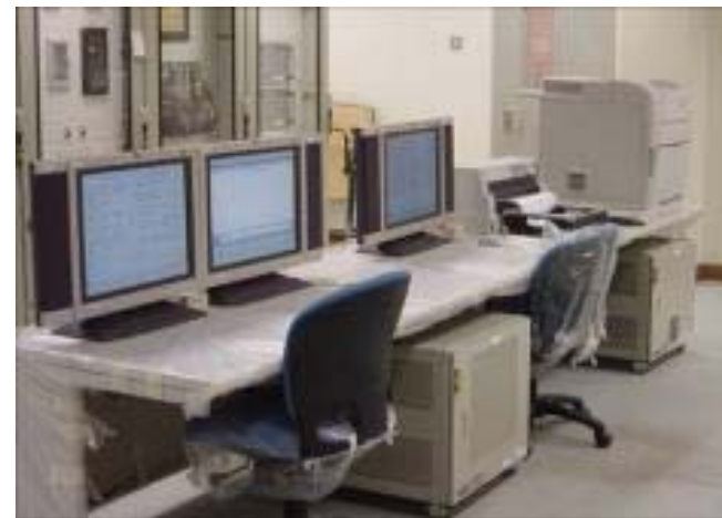
Substation Automation System
